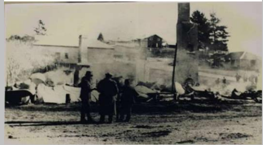
The two-storey Steampacket Hotel burnt to the ground on 25 June 1925
