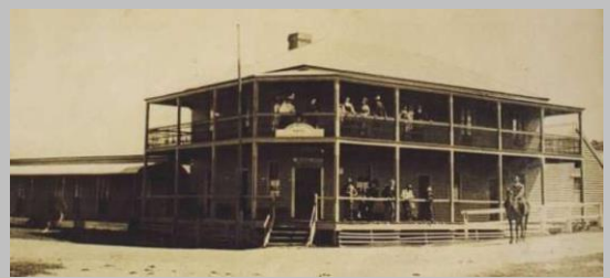
Nelligen Hotel circa 1910/16 –The first Steam Packet was built as a single-storey building in 1864. It was later renovated to double storey in 1900 so that the floor was above the height of floods. The building was destroyed by fire 1924/26.
