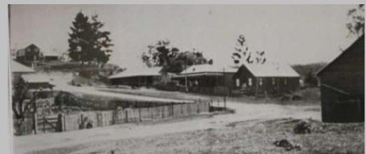
A paling fence has been erected around the former Steampacket Hotel site. The Mechanic's Institute Hall next to the post office is shown before the front was extended. The building uphill from the post office was demolished circa 1962 to widen the road that connects Braidwood St to the highway.
