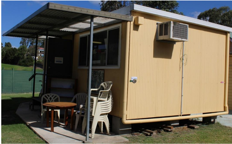
Figure 5: The Old Court House Museum's Book Emporium, housed in this demountable, is an important fund raising initiative.
